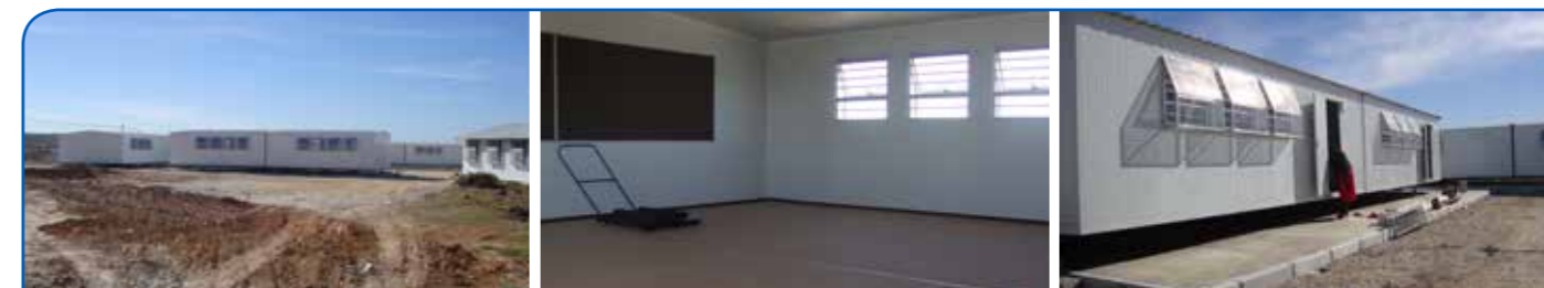
The new classrooms and paved schoolyard are due to be completed in July
